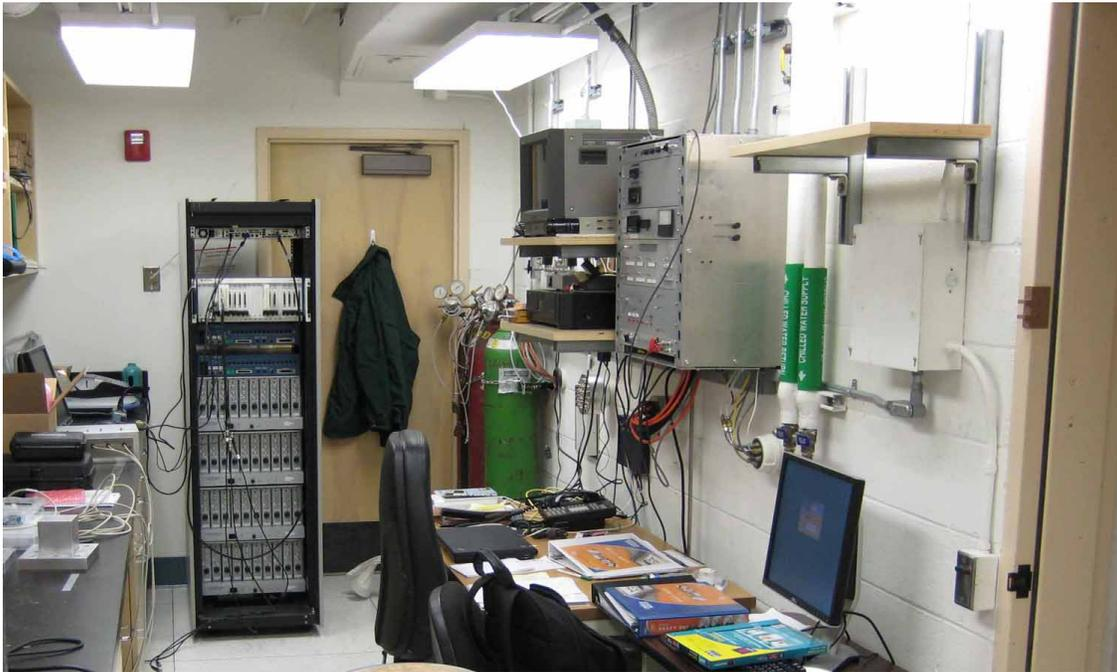
Figure 1: Control room portion of room 19 showing data acquisition system in rack panel and control system on the wall.
