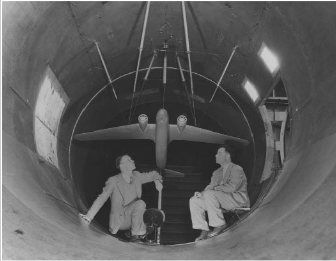
C. Millikan and Maj. Klein with DC-2 model in 10-ft tunnel.
