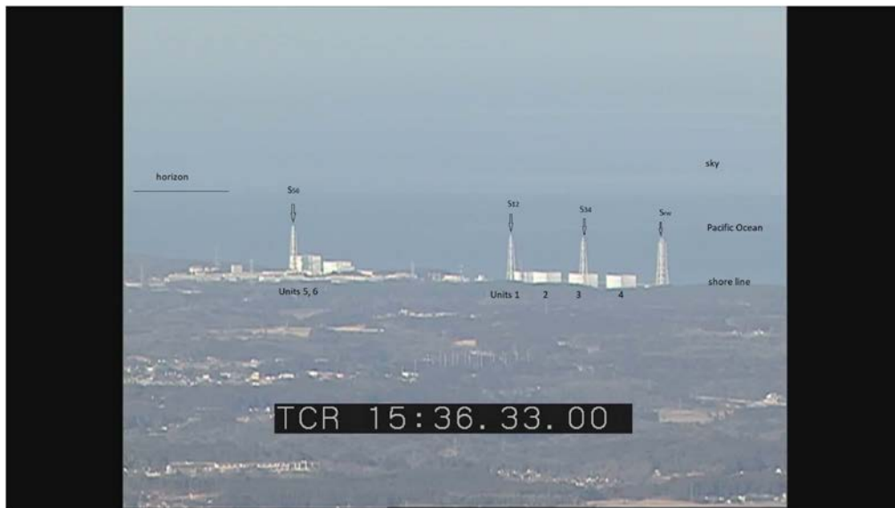
Figure 1: View of Fukushima Daiichi nuclear power plant from the FCT camera with key feature identification. Raw image of the entire frame immediately prior to the explosion event in 1F1 on March 12, 2011.
